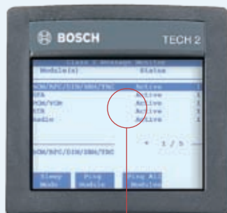
Multiplex network module status
